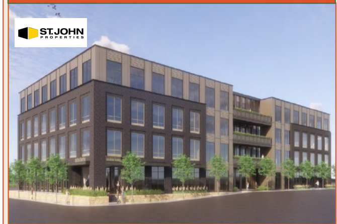
Class A Office (Block B – Pending Development)
