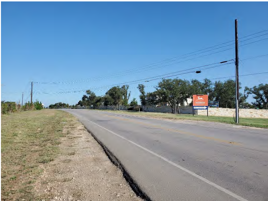
Figure 4: Southbound Approach at North Bagdad Road
