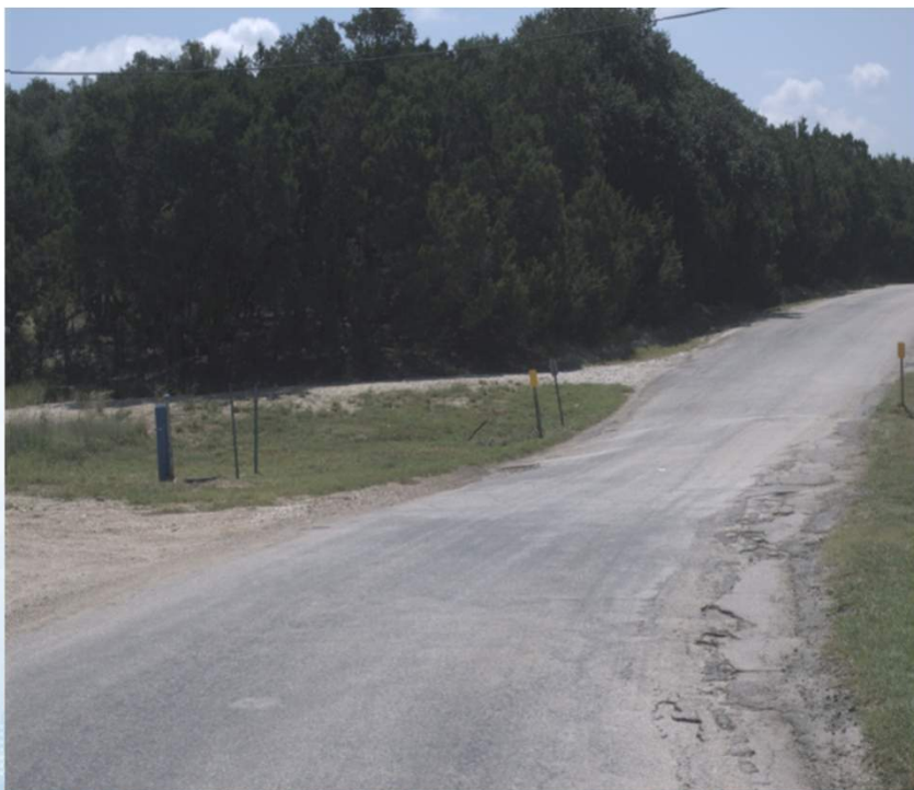
CR 270 (PCI=8.0, Failed Condition)
