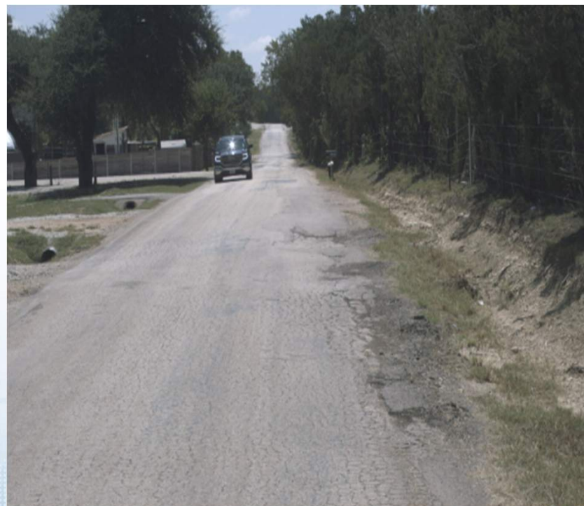
CR 270 (PCI=8.0, Failed Condition)
