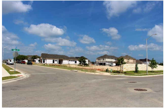
Sage Ranch Road & Stone Branch Drive
