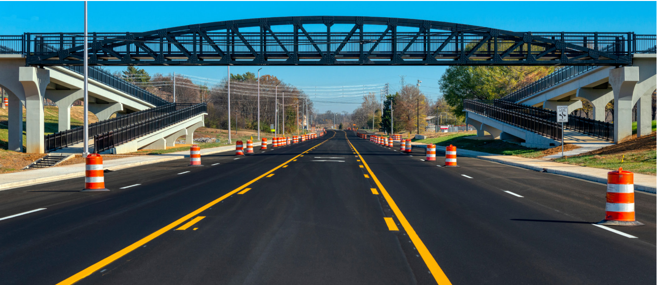
Example Pedestrian Bridge
