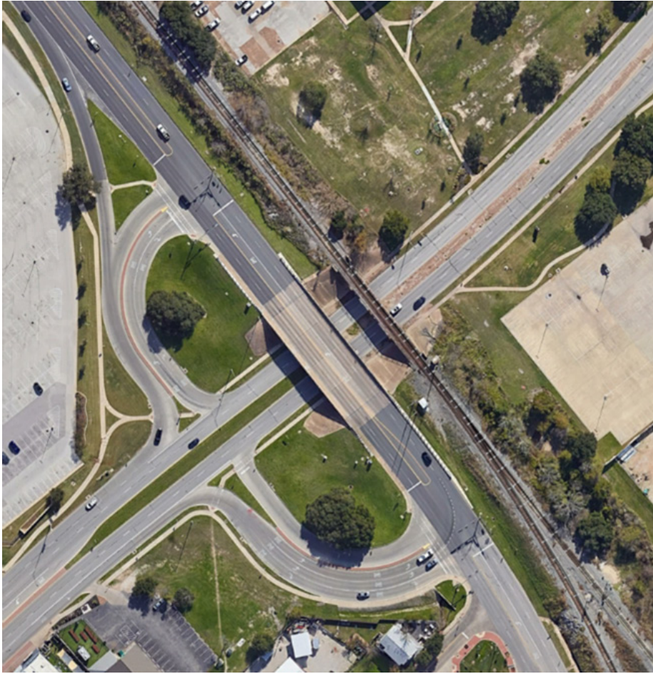
Example grade separation near a railroad
