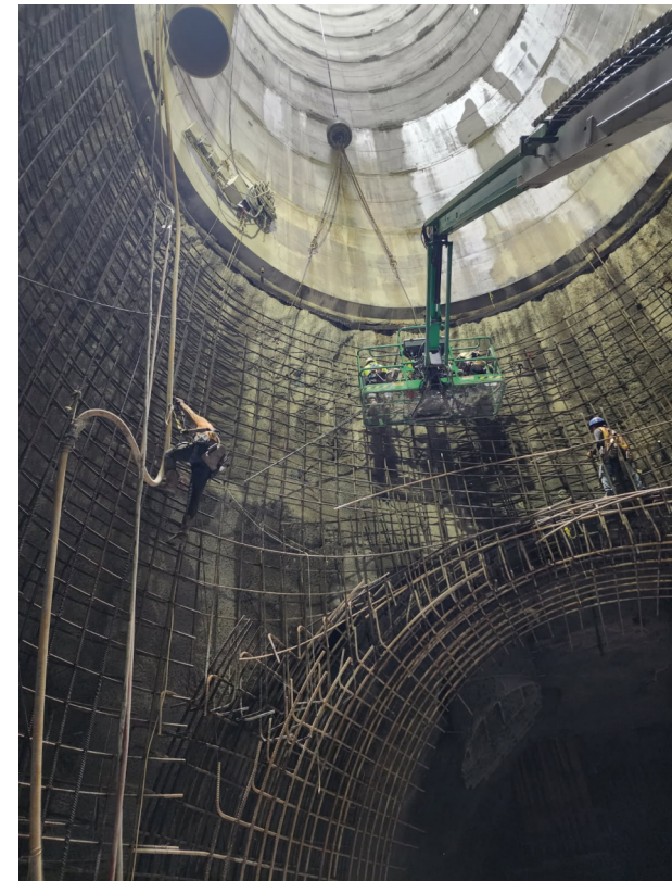
Main Shaft Rebar
