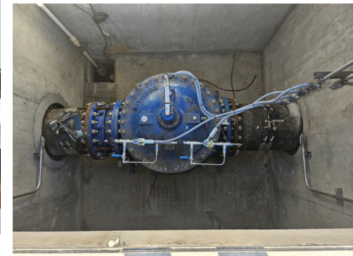
Leander Ronald Reagan Delivery Point Control Valve Modifications
