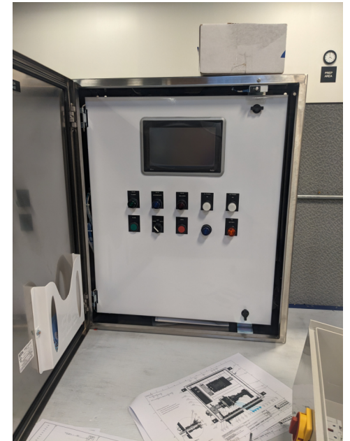
Control Panel Assembly
