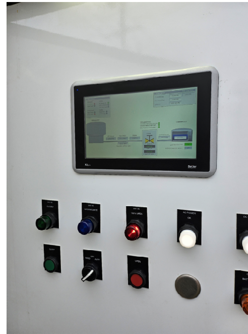
Control Panel Improvements
