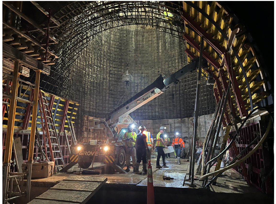
Suction Chamber Rebar and Formwork
