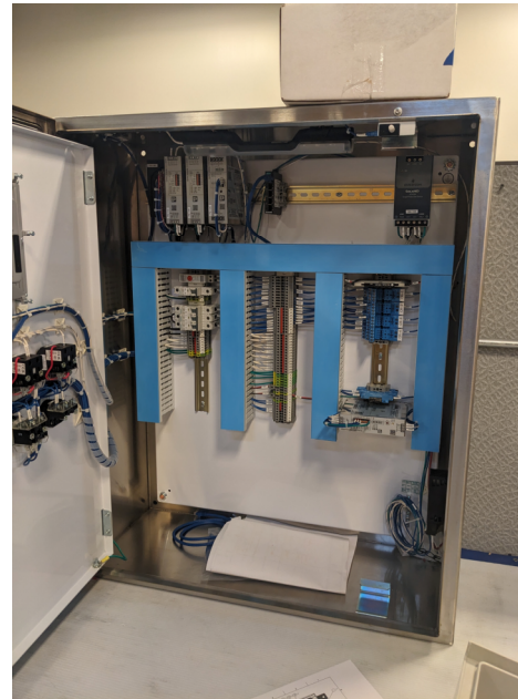
Control Panel Assembly
