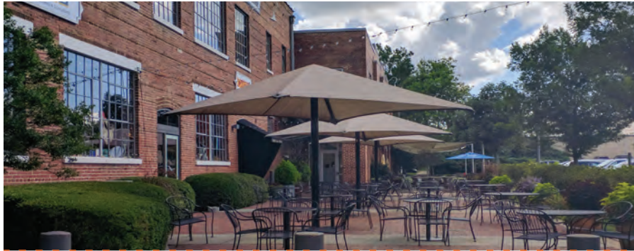
Mixed Use Building with Outdoor Seating
