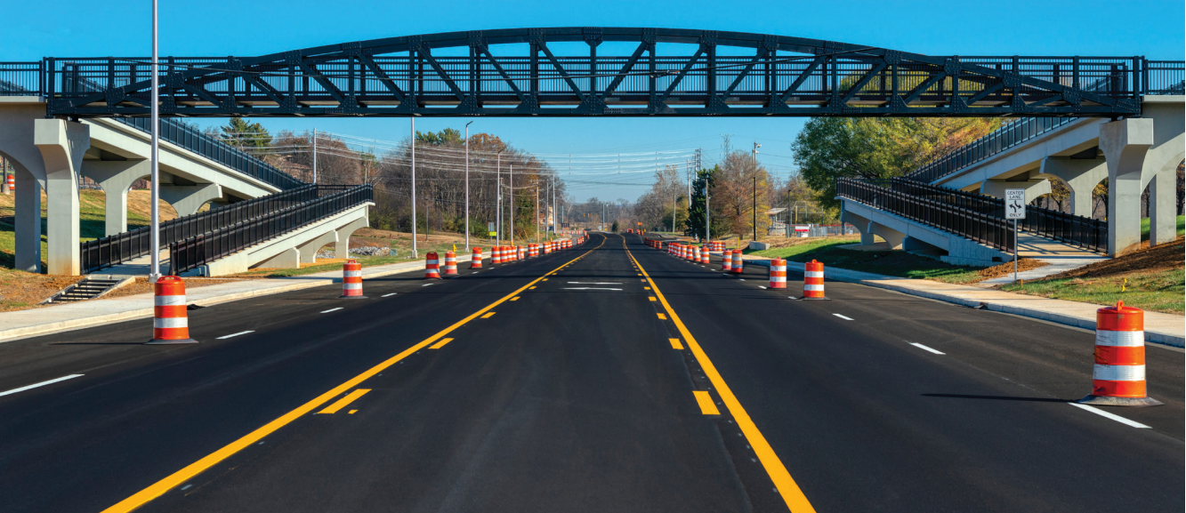
Example Pedestrian Bridge
