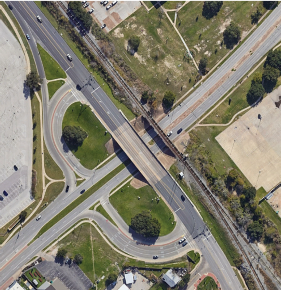
Example grade separation near a railroad
