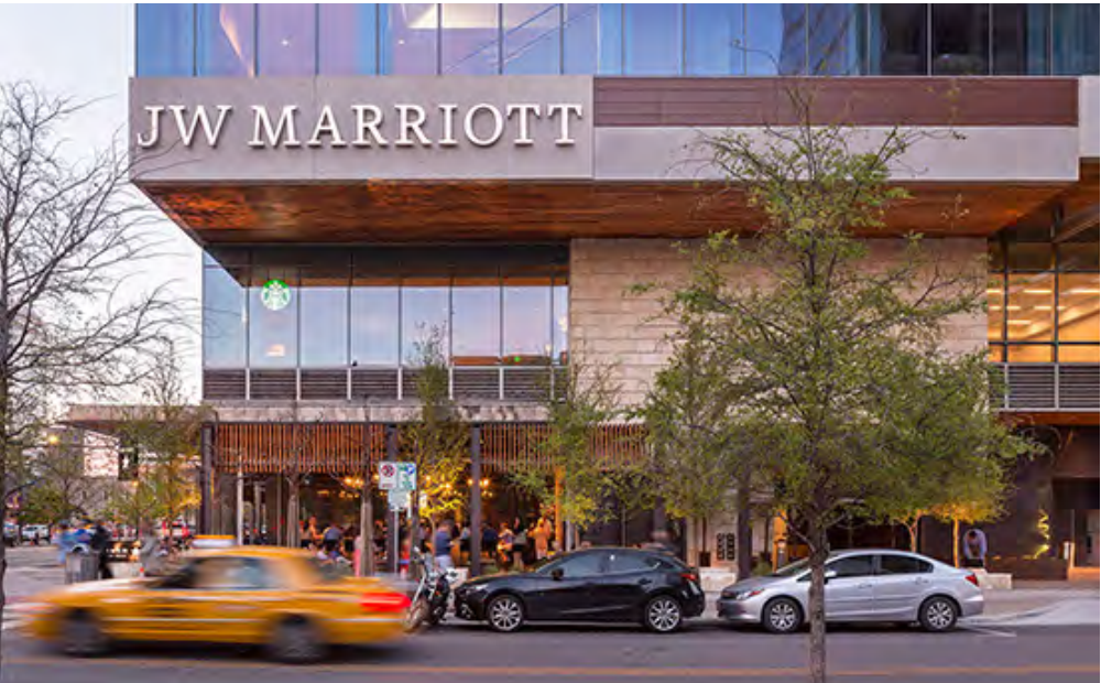
Building Identification - Wall Sign
