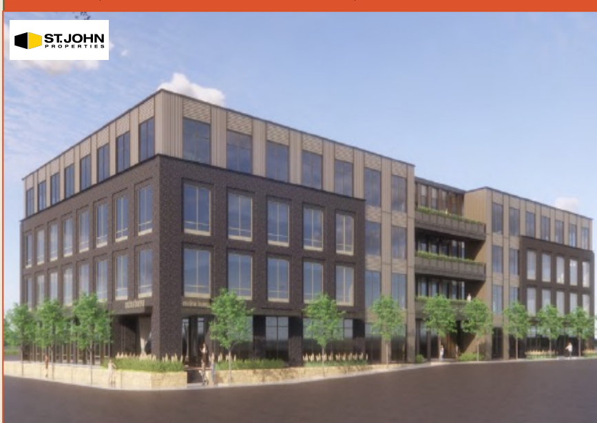
St. John Properties Class A Office (Block B – Pending Development)
